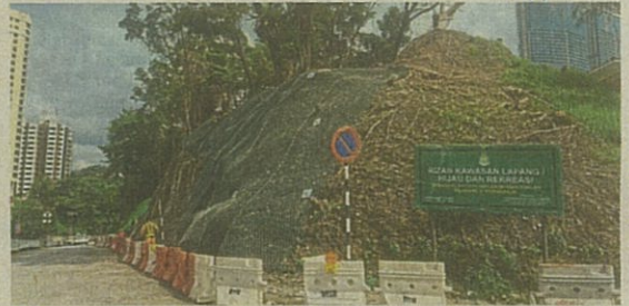
DBKL's slope enhancement project in Jalan Maarof, Bangsar. — Courtesy photo
