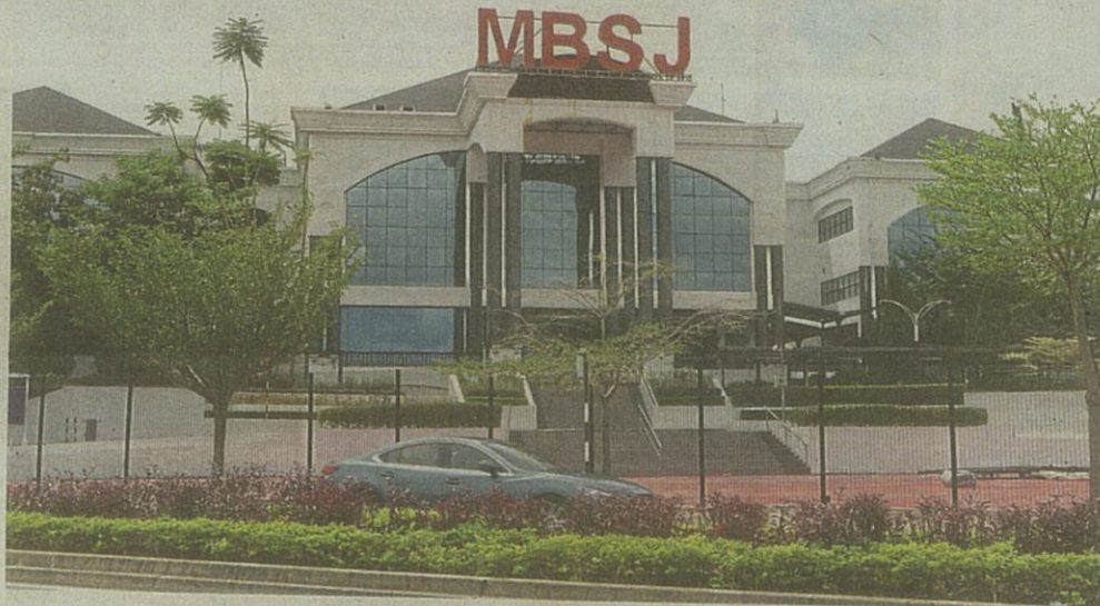
Residents want MBSJ to be more proactive and conduct inspections on the level of cleanliness and upkeep of infrastructure. — Filepic
