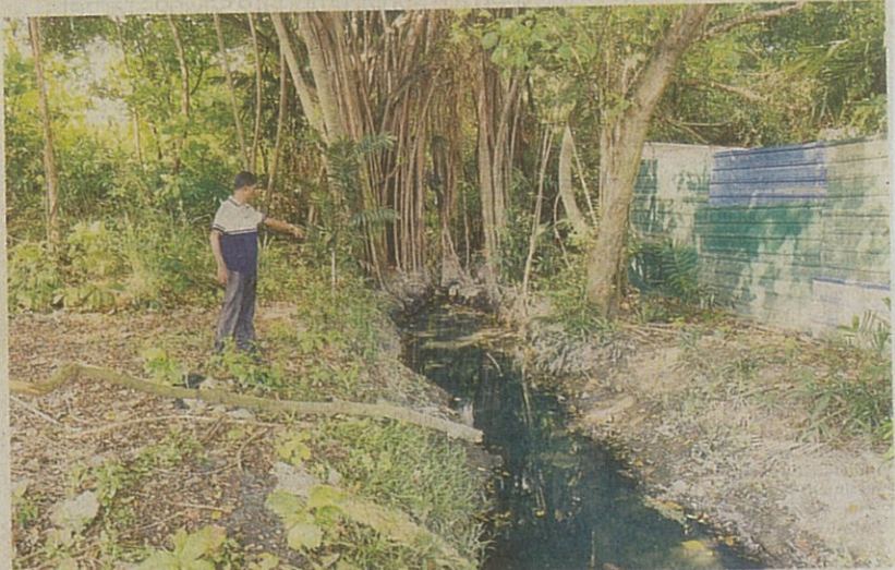
The Klang Royal City Council plans to improve drainage infrastructure in older neighbourhoods, particularly Taman Melawis, to prevent recurring flash floods. — ADIB RAWI YAHYA/THE SUN
