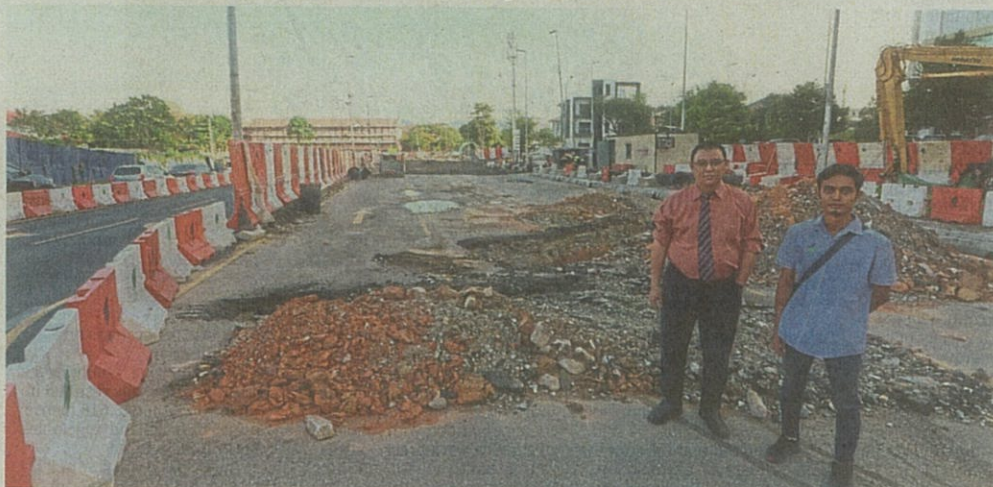
Lai (left) during his visit to the site at Jalan Sentul Pasar.
