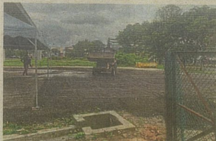
Part of the open space along Jalan Jinjang that has been paved.
