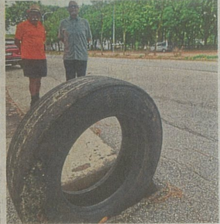
Brian (left) and Varatharajoo showing an old tyre placed in a manhole with missing cover on Jalan Delima 8 in Bandar Parklands, Klang.
