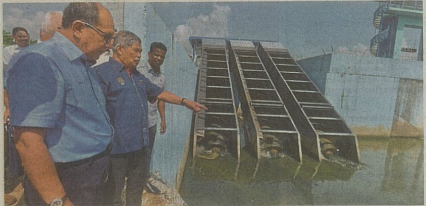
(From left) Izham and Mohamad checking out the new screw pumps at Taman Sri Muda Pump House during the launch. — RAJA FAISAL HISHAN/The Star
