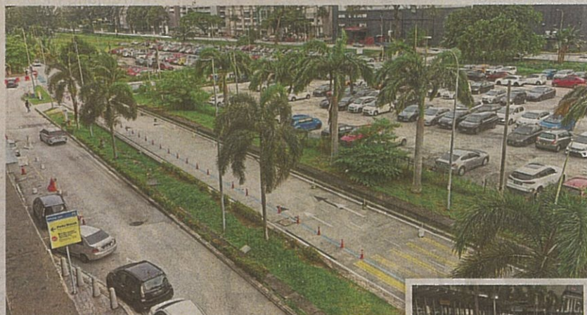
View of the bicycle lane (blue line) linking Subang Jaya LRT Station to the SS15 LRT Station. (Inset) The 4,303m-long bicycle lane that was completed within two months. — Courtesy photos
