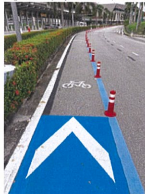
The 4,303m-long bicycle lane that was completed within two months. — Courtesy photos
