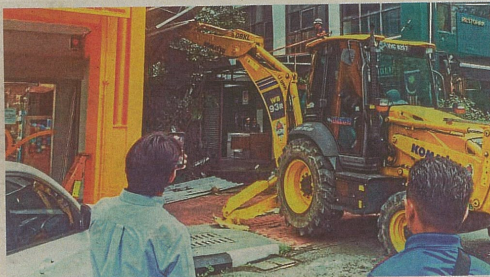
(Left) Illegal extensions in lanes along Jalan Medan Setia 1 being demolished.
