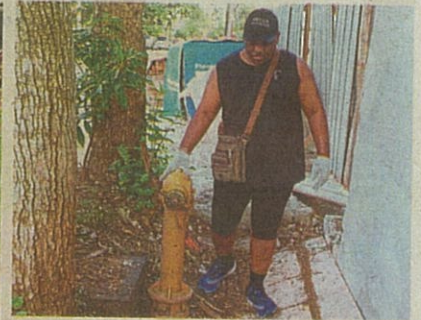
Alvin often finds hydrants hidden by illegal structures, parked cars and overgrown vegetation.
