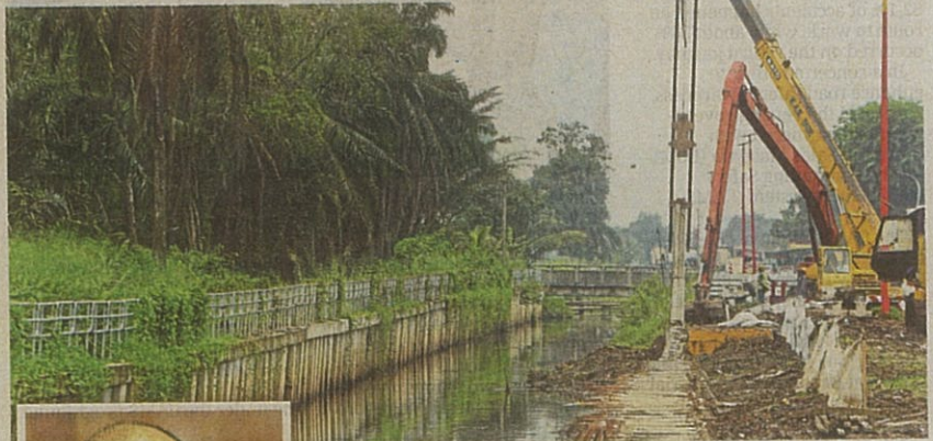
Flood mitigation works along Sungai Kandas in Klang is one of the 32 projects under DID. — KK SHAM/The Star
