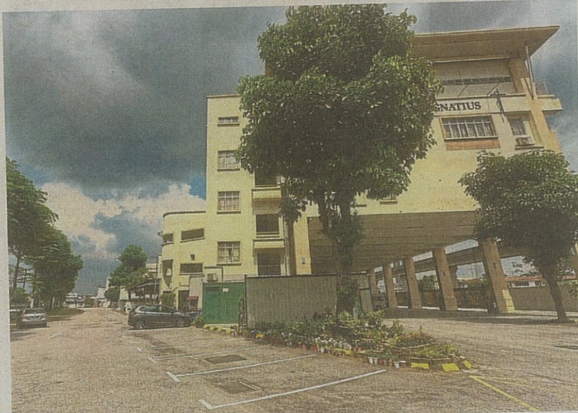
To the left is the St Ignatius Church carpark along Sungai Kayu Ara where ongoing flood mitigation works are taking place.
