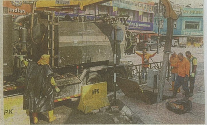
MBDK's Environmental Services Department cleaning crew removing fats, oil and grease from a sump in Klang's Little India. — KK SHAM/ The Star
