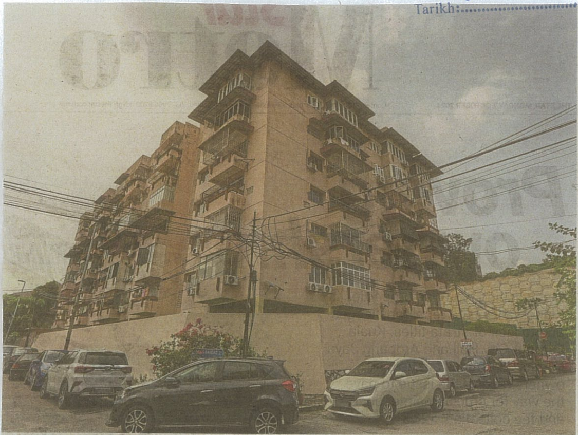
Fairview Mansion in Taman Desa was built in 1979 and much of its infrastructure is ageing and in dire need of replacement. — Photos: YAP CHEE HONG/The Star
