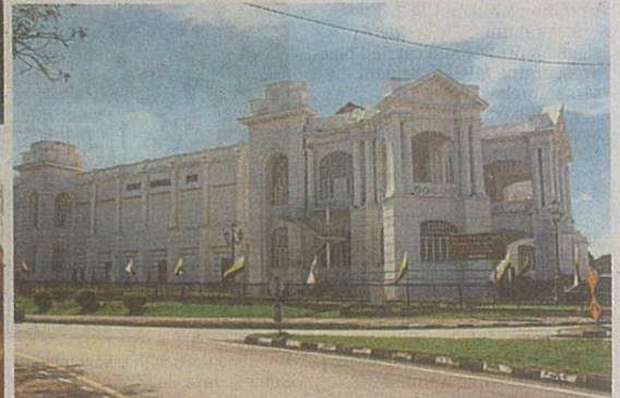
Ipoh Town Hall building reflects the city's colonial past.
