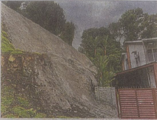
Remedial works on a slope along Jalan Melawati 3, Taman Melawati have been completed following soil erosion in May.
