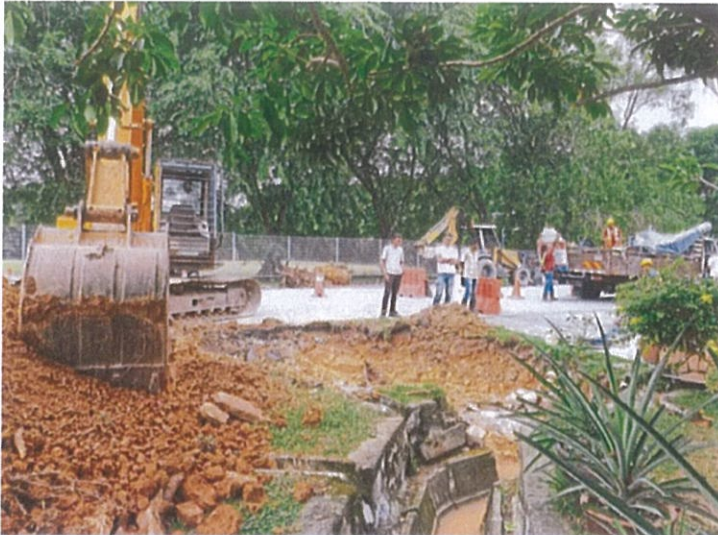
Workers carrying out earth works at the Jalan SS14/7C intersection to build a scupper drain.
