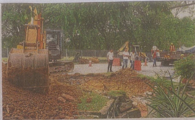
Workers carrying out earth works at the Jalan SS14/7C intersection to build a scupper drain. 9 Apr 9/7 (MBSJ)
