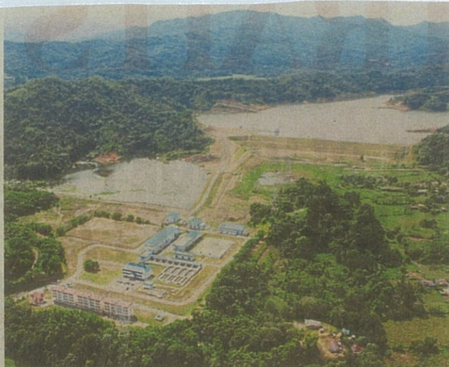
The capacity at the Telibong II Water Treatment Plant in Sabah will be expanded this year.
