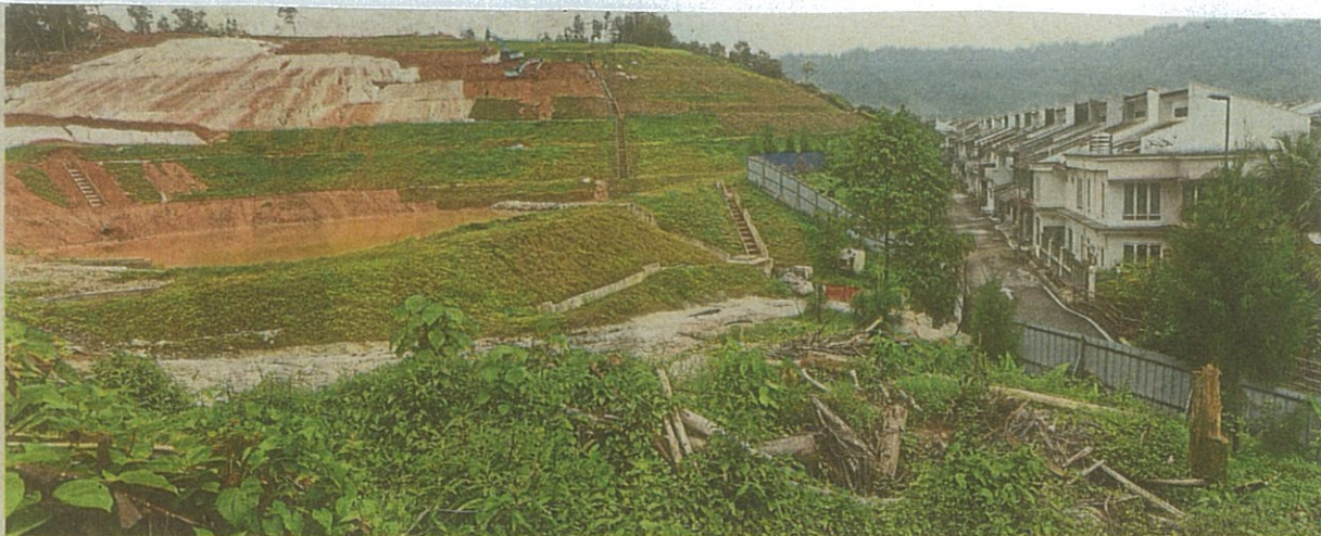
Residents are worried over slope stabilisation works next to Taman Sering Ukay in Bukit Antarabangsa. — Photos: LOW BOON TAT/The Star
