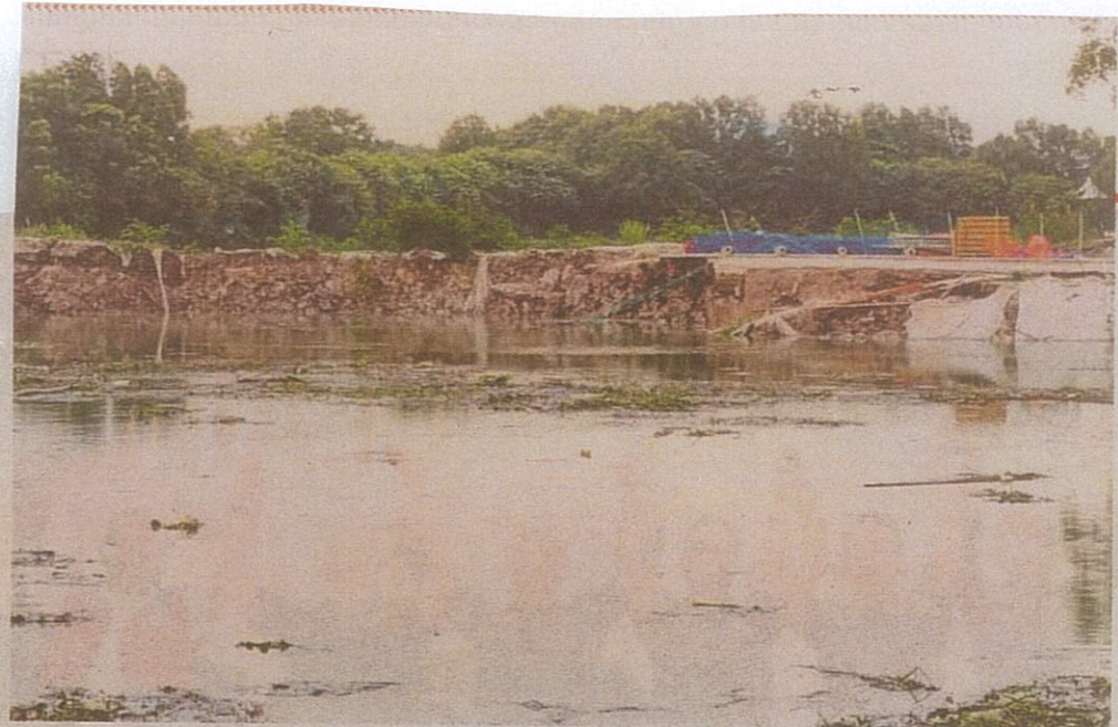
A pond embankment collapsed following a landslide near Idaman BSP in Taman Mas, Puchong, on Saturday.
