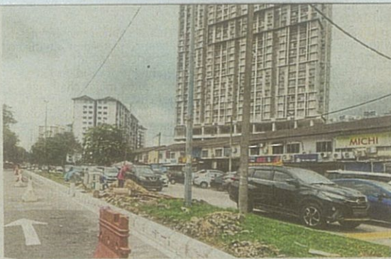
The road kerb at Jalan Langkawi is being upgraded, says Lai.
