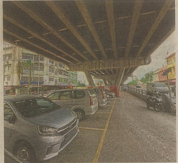
The mechanical parking bay project under the Jalan Yew-Jalan Sungai Besi flyover is awaiting DBKL's approval. — LOW BOON TAT/The Star
