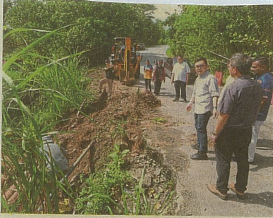
Chua (third from right) checking on the progress of the bridge upgrading works.
