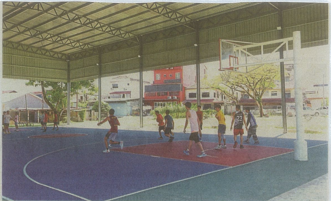
Regardless of the weather, youths can play basketball at the new covered court along Jalan 13/32 in Jinjang Selatan. — Photos: LOW LAY PHON, LOW BOON TAT/The Star
