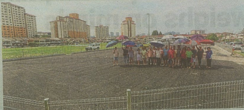
Taman Indah Perdana residents claim that the parking space built by MPS is inadequate to accommodate the number of vehicles in the neighbourhood. — CHAN TAK KONG/The Star
