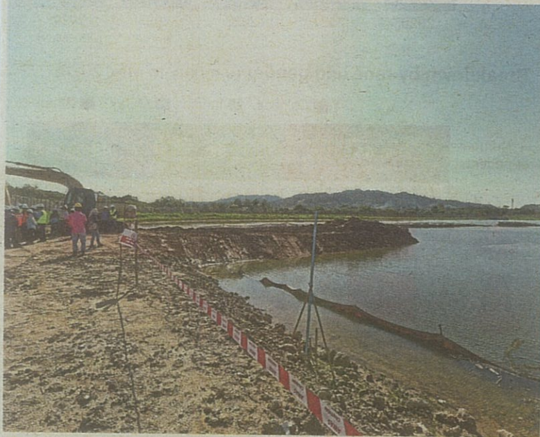
Package D of the Water Resources Assurance Scheme in Jenderam Hilir is facing a 6.23% delay. — Filepic
