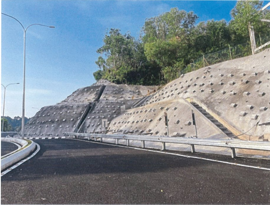
The new connecting road between Kinrara Industrial Park and Jalan BK 5B Puchong.
