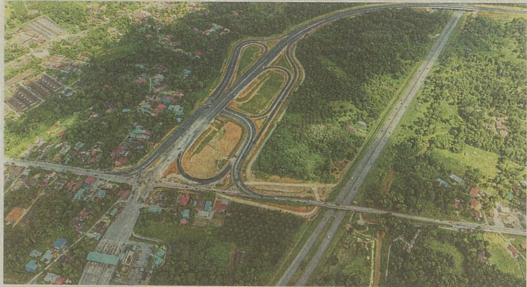
New way: An aerial view of Section 11 of the WCE, covering the route between the Taiping Selatan and Beruas elevated interchanges.
