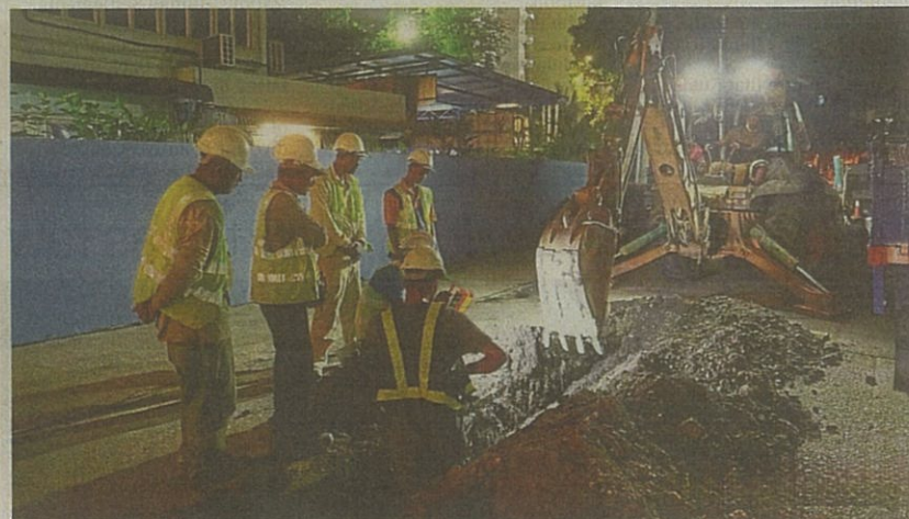
DBKL enforcement team carrying out a spot check at a construction site in downtown Kuala Lumpur. — Courtesy photo
