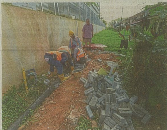
Contractors laying out water pipes in a housing area in Seri Petaling.
