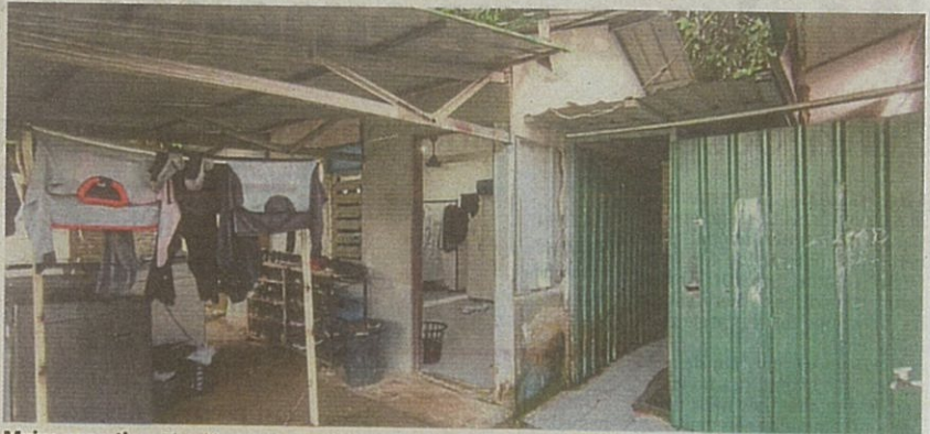
Major operation: The dilapidated conditions in one of the 20 homes that were raided in Selangor and Negri Sembilan.
