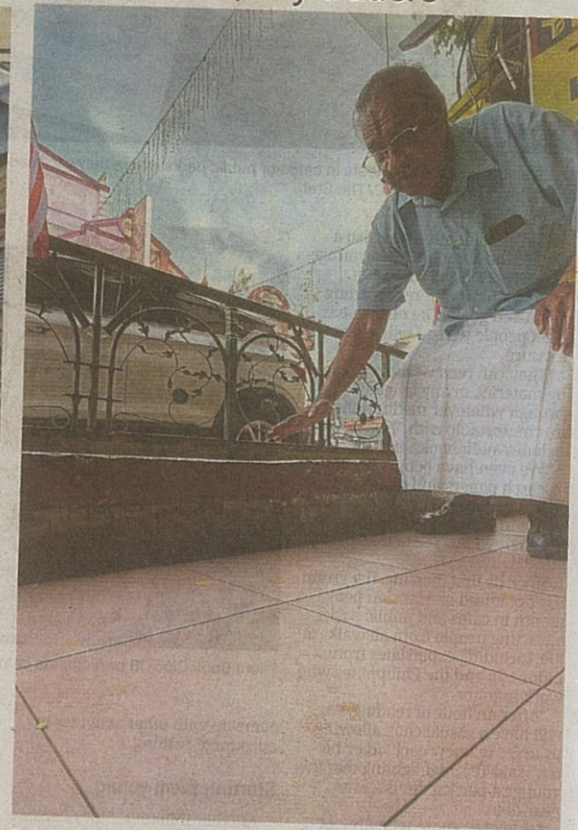
Raman showing how high the water rises when it rains heavily, inundating shophots along Jalan Tengku Kelana in Klang's Little India. — LOW BOON TAT/The Star
