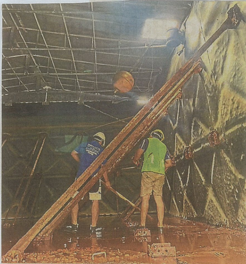
The bottom of a water storage tank filled with sedimentation.
