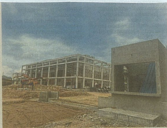
Construction work is ongoing at MBSJ's multipurpose sports complex in Pusat Bandar Puchong.
