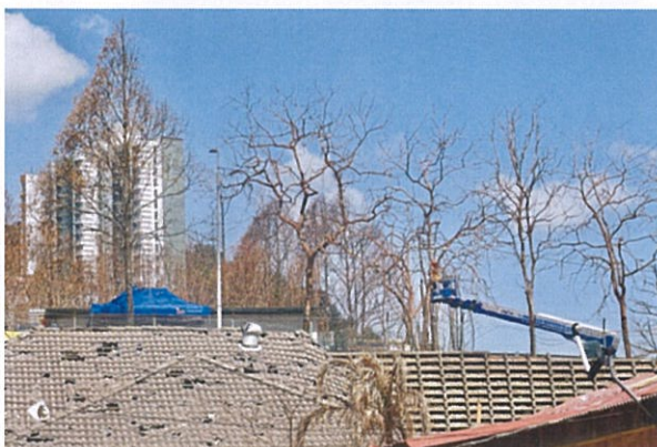
Ongoing operation: Workers felling burnt trees at Kampung Kuala Sungai Baru.
