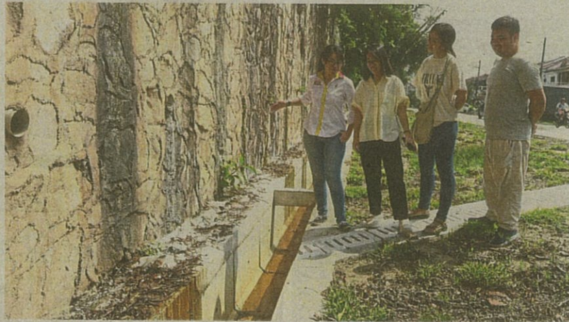
(From left) Wong and Suzanah at the site of the newly upgraded drain along Jalan BS 3/1 in Bukit Serdang, Seri Kembangan. With them are staff from Wong's office.
