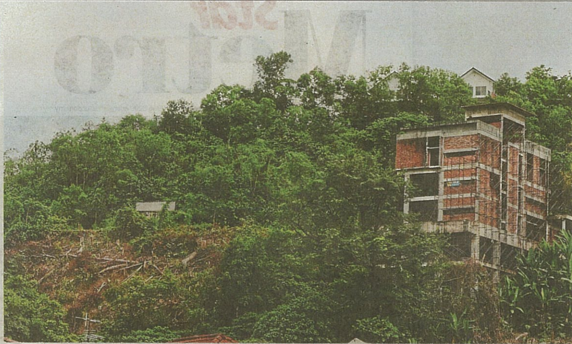
Hill slope development in places like Taman Melawati in Hulu Kelang is cause for concern among nearby residents. — AZMAN GHANI/The Star
