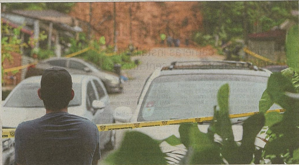
File photo of residents looking at the site of the landslide-hit area at Jalan E6 in Taman Melawati.
