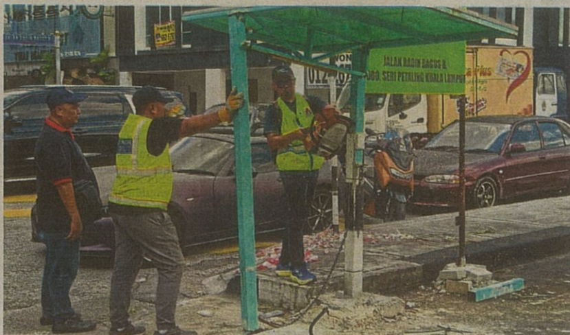
DBKL officers removing structures built by parking touts at Jalan Radin Bagus 8.
