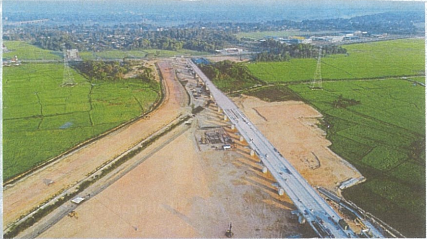
The East Coast Rail Link project in progress in Kelantan last month. The Malaysian Investment Development Authority says companies can tap sectors such as construction and renewable energy along the East Coast alignment. PIC BY NIK ABULLAH NIK OMAR
