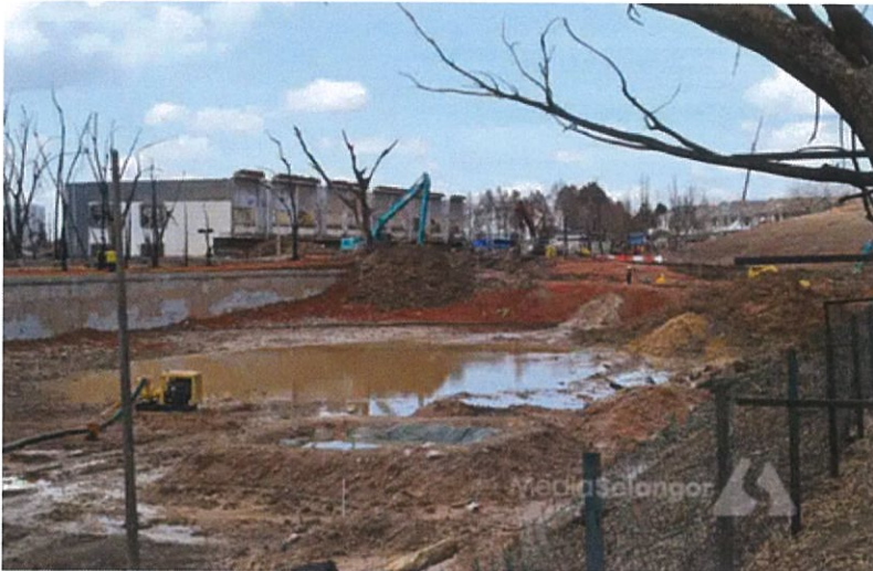
A view of the crater left behind by the April 1 gas pipeline fire, as seen in Putra Heights, Subang Jaya on April 12, 2025. — Picture by HARUN TAJUDIN/MEDIA SELANGOR
