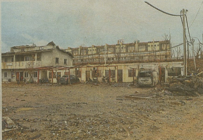
Critical issues: Houses damaged in the gas pipeline fire, which has raised pressing legal questions about preparedness, accountability structures and regulatory safeguards in Malaysia when industrial disasters occur. — MUHAMAD SHAHRIL ROSLI/The Star
