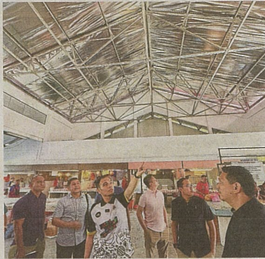
Syahredzan (fifth from left) showing the newly installed roof at the market. — SHAARI CHEMAT/The Star
