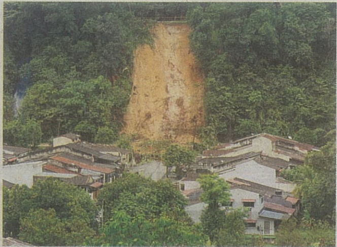
The landslide in Taman Melawati has caused 20 terrace houses to be cut off from the main road. — ADIB RAWI YAHYA / THE SUN
