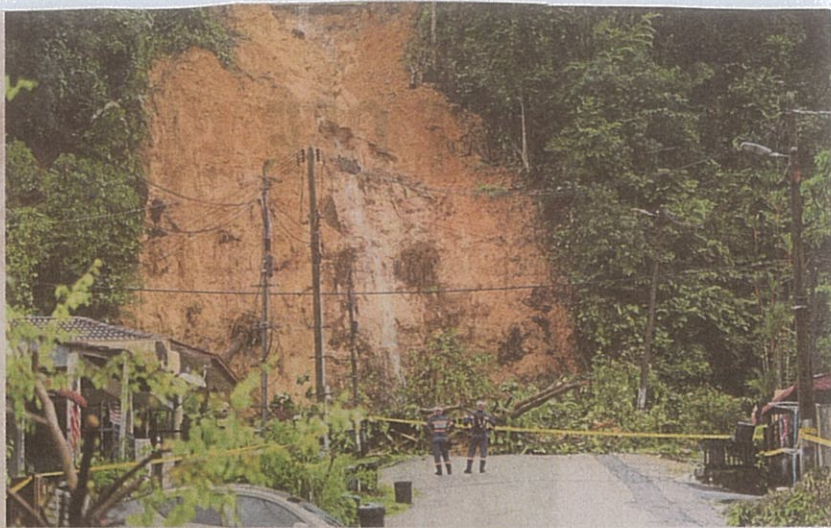
The area where a landslide happened in Taman Melawati yesterday.
