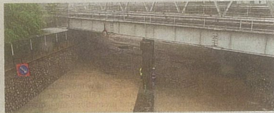
Flash flood at Jalan Chan Sow Lin, Kuala Lumpur. — DBKL Kuala Lumpur Command and Control Centre Facebook page.
