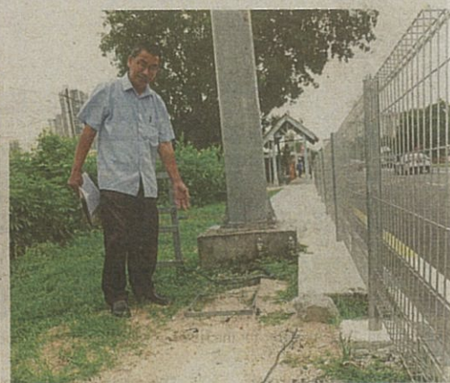
Yee showing exposed wires which could endanger passers-by at the residential area.
