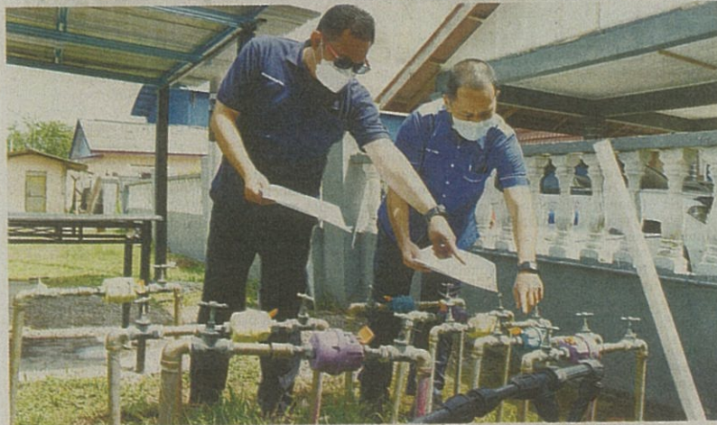
In the event of a dispute, Air Selangor will monitor the customer's water trends using a 'smart meter' for three consecutive days to establish the possibility of internal leakage in the water pipe. —BERNAMAPIC
