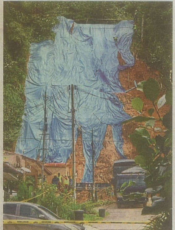
Workers placing tarpaulin sheets on the affected hill slope in Taman Melawati in Hulu Kelang, Selangor. — SHAARI CHEMAT/The Star
