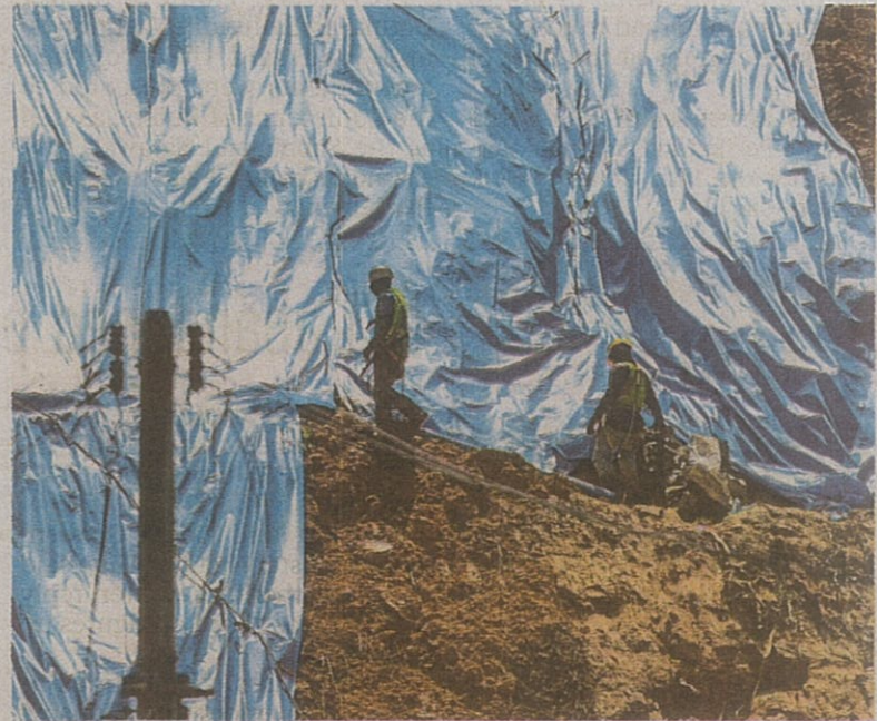
Contractors installing tarpaulin sheets to protect the exposed topsoil in Ampang yesterday. PIC BY ASWADI ALIAS
