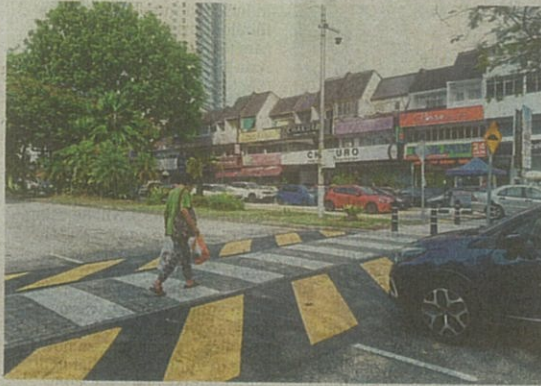
The raised pedestrian crossing in Jalan Tun Mohd Fuad, TTDI has helped in slowing down cars.
