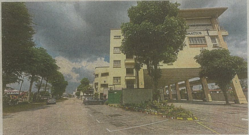
A view of St Ignatius Church's carpark and Sungai Kayu Ara (left, beyond the fence) where flood mitigation works are being carried out. — Filepic
