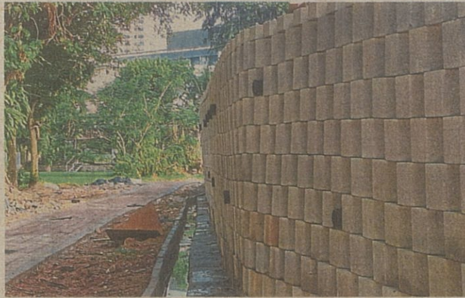
The retaining wall at the Astaka field is leaning forward slightly. (Right) Some of the bricks used to construct the retaining wall are already broken.
