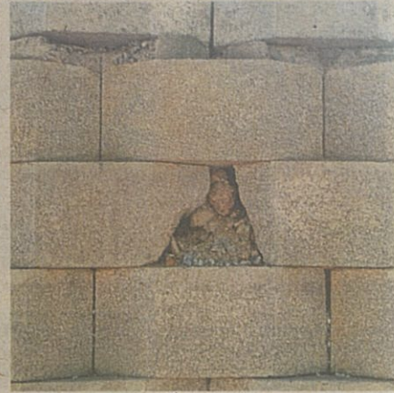
The retaining wall at the Astaka field is leaning forward slightly. (Right) Some of the bricks used to construct the retaining wall are already broken.
