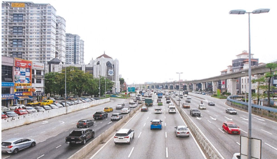
Flood mitigation upgrading works near IOI Mall Puchong have been delayed, due to pipe realignment works passing beneath the LDP highway. — MUHAMAD SHAHRIL ROSLI/The Star
