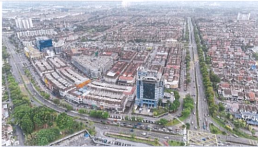
Aerial view of USJ5 showing a mix of residential and commercial areas. — Photos: IZZRAFIQ ALIAS/The Star
