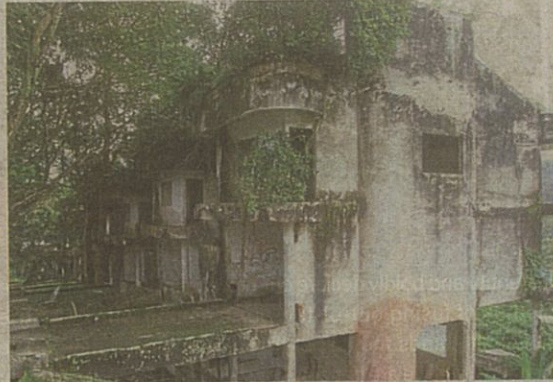
Long way to go: Nga said the restoration of abandoned projects takes between one and five years, subject to the complexities of the projects.
