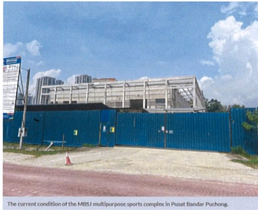
The current condition of the MBSJ multipurpose sports complex in Pusat Bandar Puchong.
