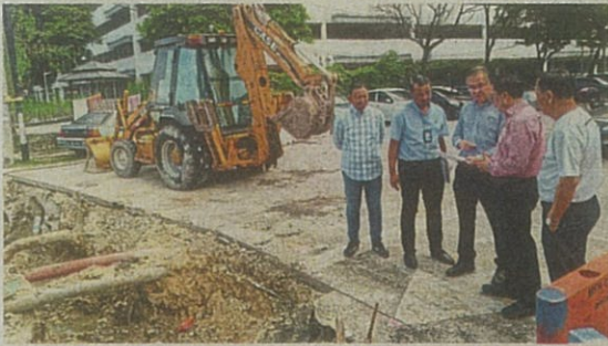
(From second right) Mohd Kamri with Yap and other representatives during the site visit to check on the progress of a drain upgrading project in Kampung Baru Ampang.
