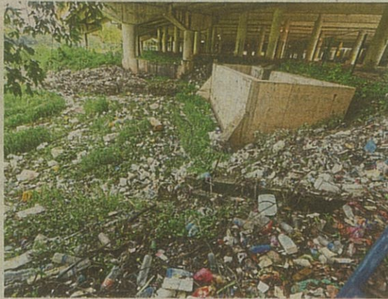
The Taman Midah flood retention pond is an eyesore with rubbish scattered all over the place. — Filepic
