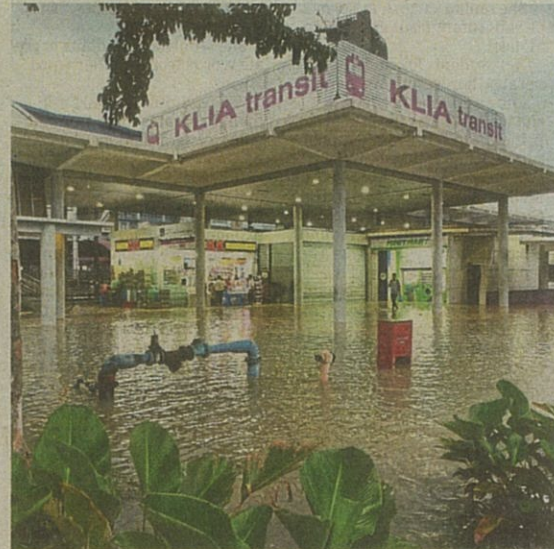
TBS transit hub, located beside the flood retention pond, inundated with floodwaters recently. — Filepic
