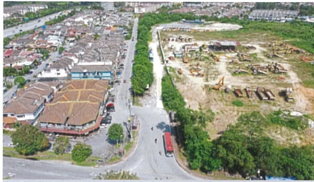
The proposed Jalan TK5/32 (marked in red) is an access road built specially for the Taman Kinrara Section 5 area. — Photos: IZZRAFIQ ALIAS/The Star
