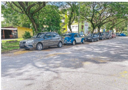
The speed bump at Jalan TK4/5 near Pangsapuri Ceria is barely visible.
