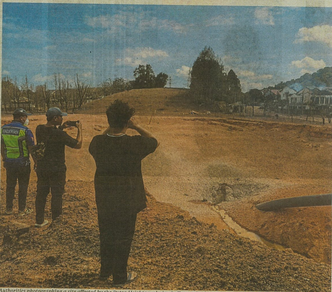
Authorities photographing a site affected by the Putra Heights explosion in Taman Puchong Perdana, Selangor, yesterday. BERNAMA PIC
