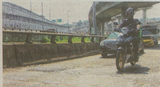
RM33,000 has been allocated to repair the flyover joint, which is expected to take four weeks. — MUHAMAD SHAHRIL ROSLI/The Star
