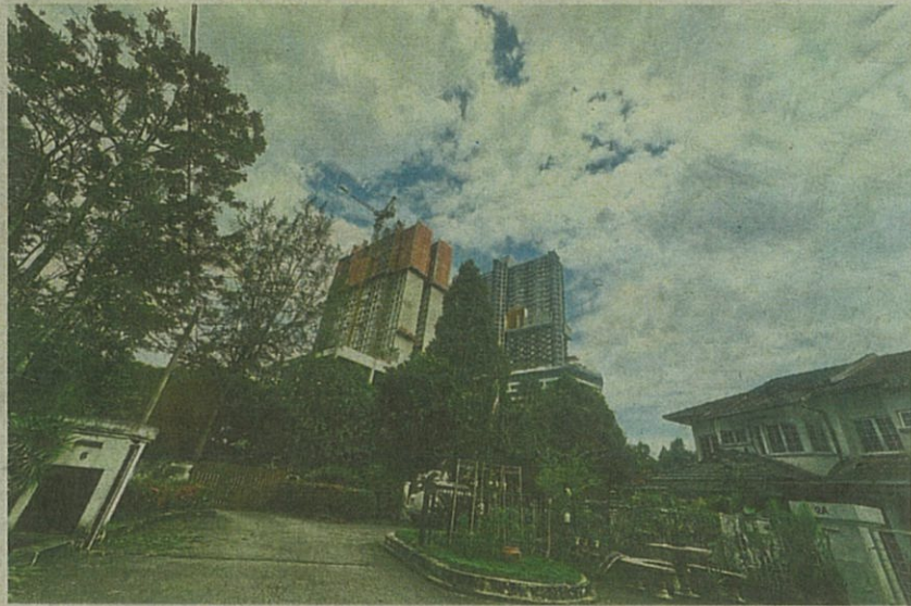
More projects near or on slopes are giving locals cause for concern. — Photos: LOW LAY PHON and IZZRAFIQ ALIAS/The Star
