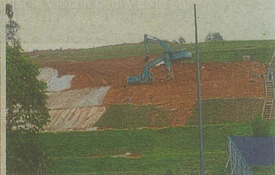
MPAJ is undertaking works to stabilise the slopes in Taman Sering Ukay. — Filepic
