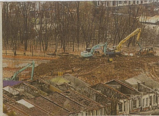
Restoration work being carried out at the site of the Putra Heights gas pipeline fire in Subang Jaya on Monday. NSTP PIC BY EIZAIRI SHAMSUDIN
