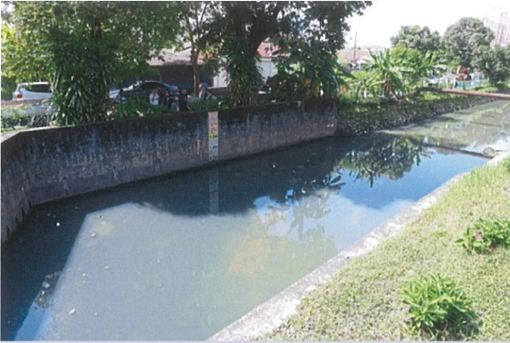
The anti-flood wall along Jalan TK 2/11 is being lengthened by 185m.
